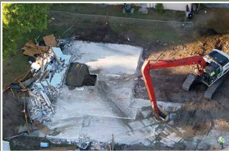
This aerial photo shows workers picking up remnants from a home in Seffner, Fla. A huge sinkhole opened under the bedroom in this home and swallowed the owner, Jeff Bush.
